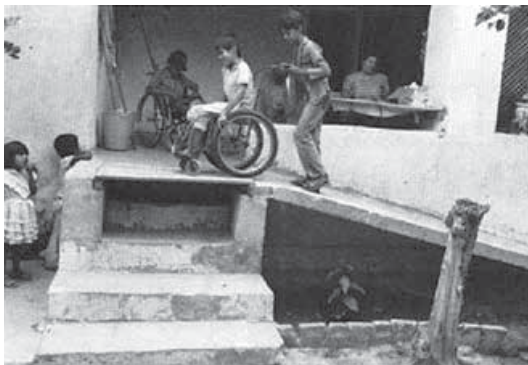
The health workers of Project Piaxtla built this ramp so the wheelchair riders could come into the clinic more easily. (Photo: John Fago)
