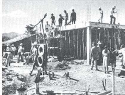
Villagers and visiting students building the PROJIMO workshop.
