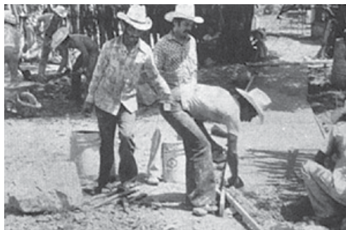
In the village of Ajoja, Mexico, over 60 families participated in building a cement walkway from the rehabilitation center to the main street.
