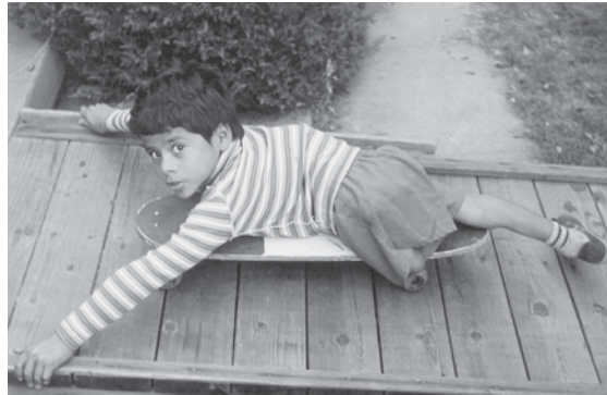
A narrow wood ramp with sideboards lets this child pull himself up it on his skateboard.
